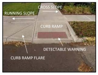
**Detectable Warning:** Surface consisting of truncated domes aligned in a square or a radial grid pattern, and built in or applied to a walking surface.
