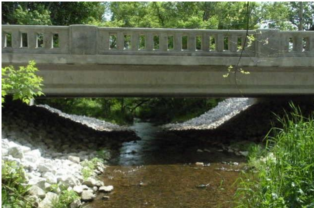
Alden Road Bridge - Alden, IL
