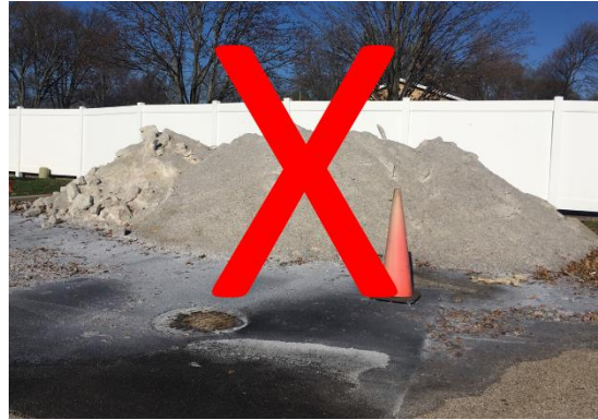
Improperly stored salt pile
