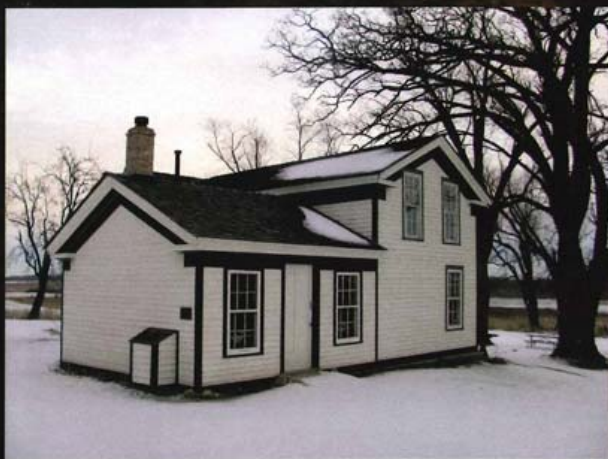
Powers-Walker Historic Site, Ringwood
