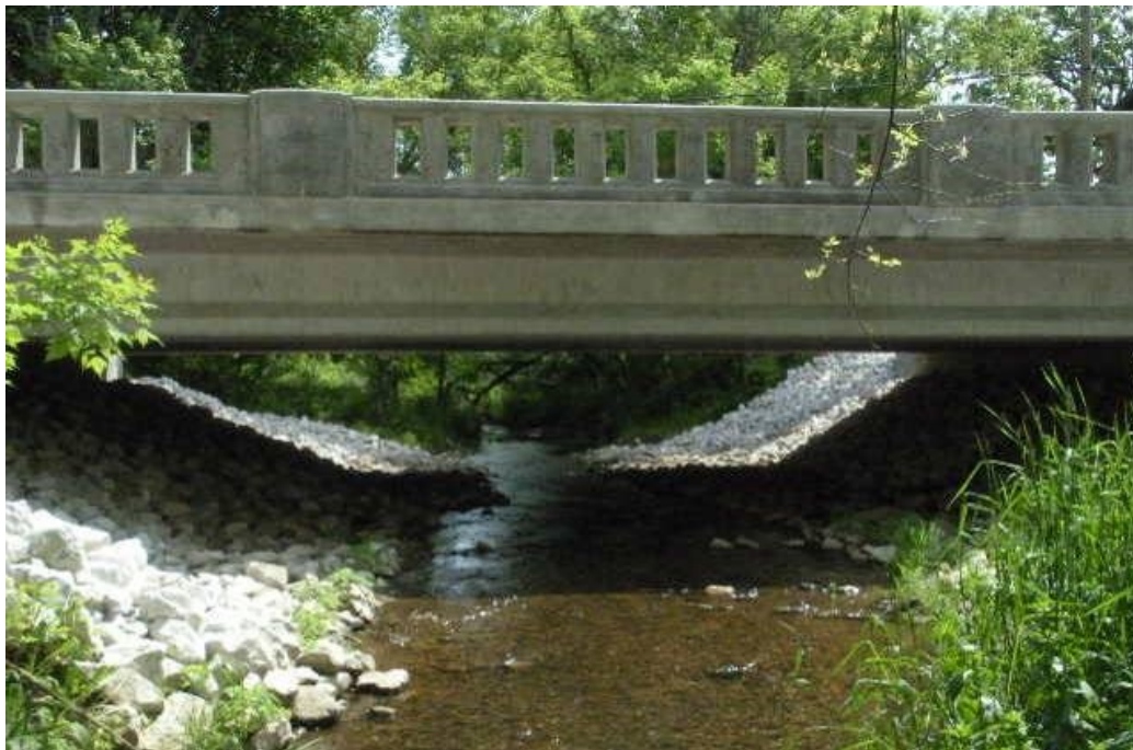
Alden Road Bridge - Alden, IL
