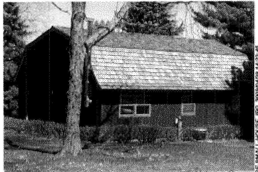
SHED CONVERTED INTO SMALLER CARETAKER QUARTERS
