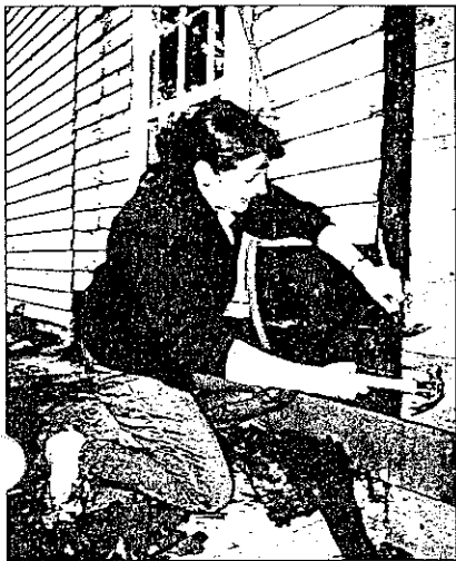
Gail Drabant removes 1850 siding from the Powers-Walker House for reuse later.
