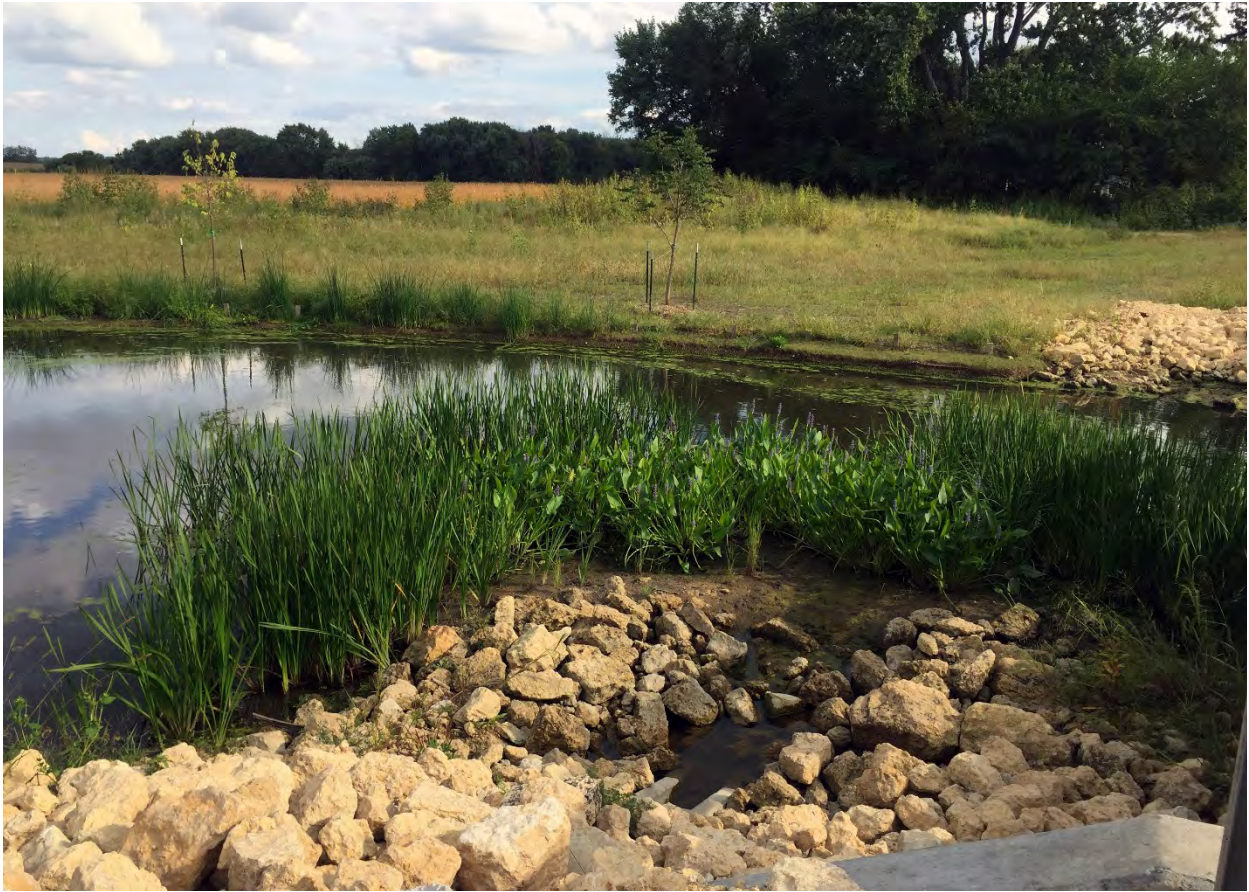
The new channel and plug plantings.
