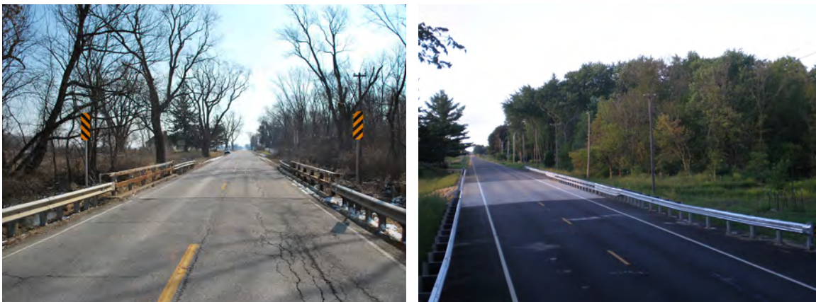
Looking south, a dramatic transformation from existing condition to final construction.
