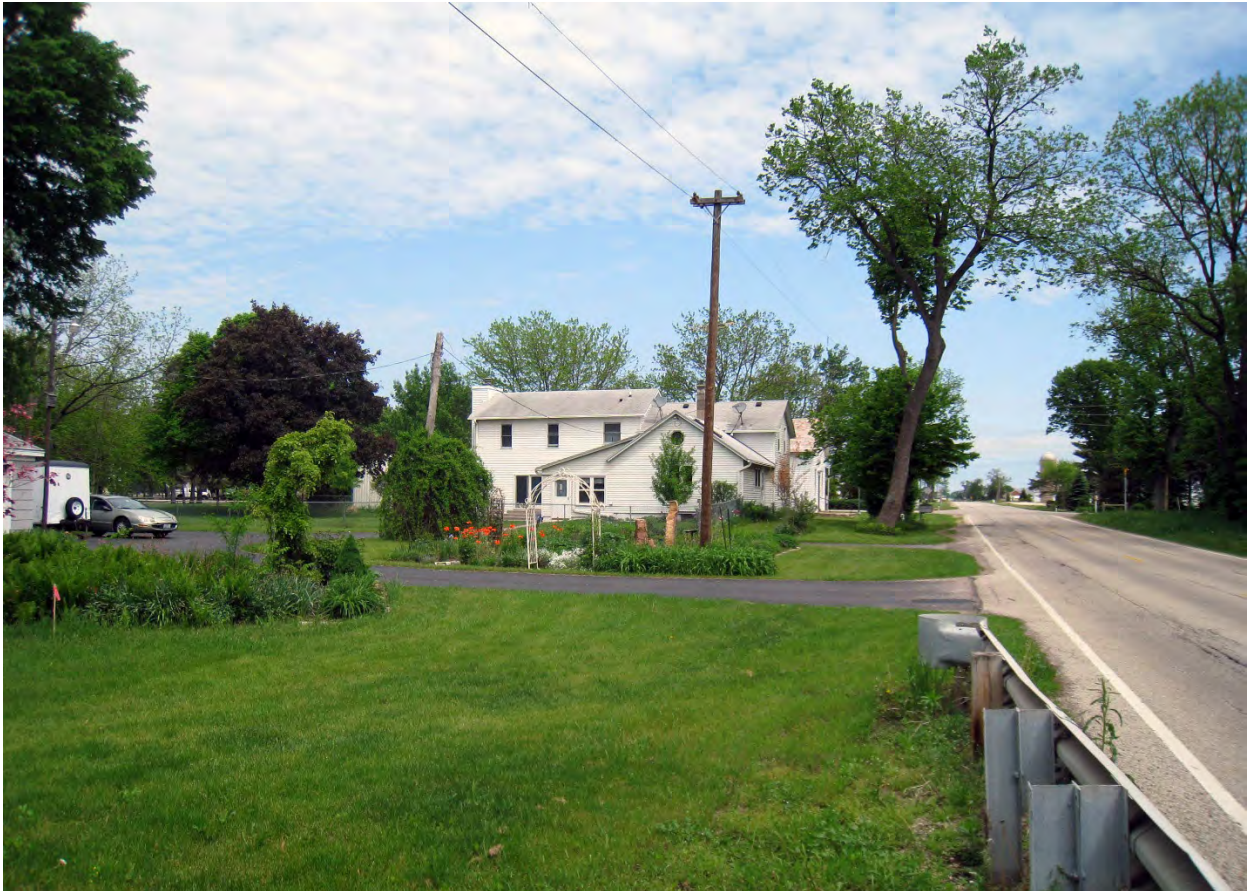
The Blue's home is located at the edge of the existing right-of-way, limiting the opportunity to modify the roadway profile.
