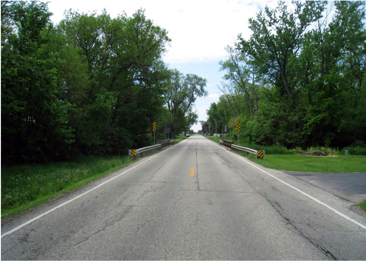
Looking south, the existing roadway corridor prior to construction.
