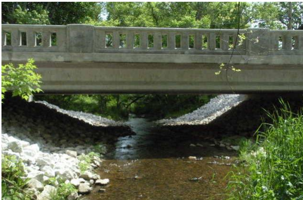
Alden Road Bridge - Alden, IL
