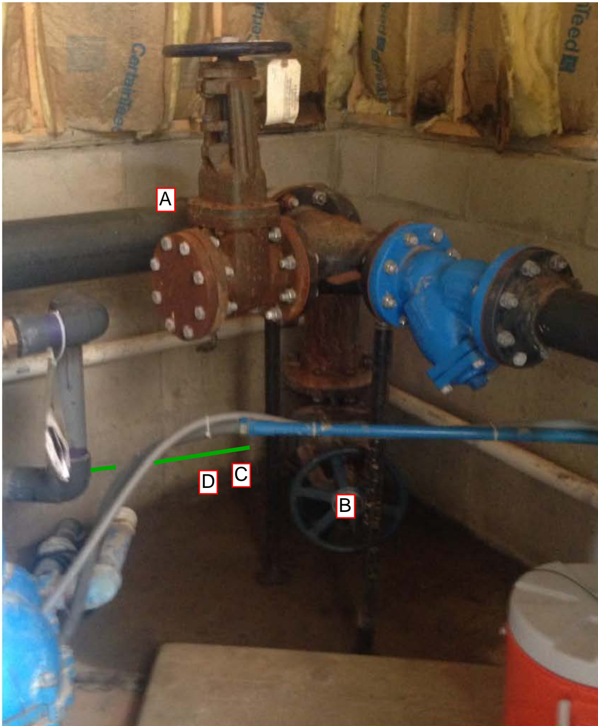
Piping Work – Valley Hi Well house #2
