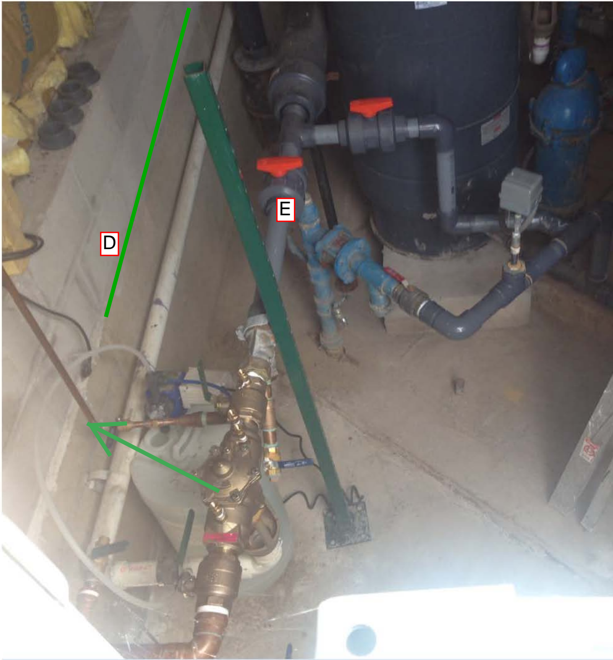
Piping Work – Valley Hi Well house #2
