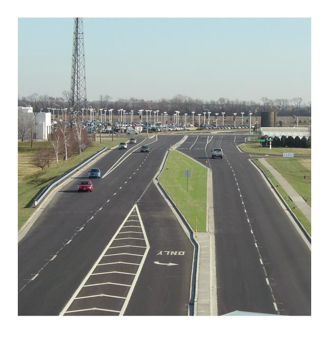
Patrick and BLA succeeded in helping MCDOT to increase the safety and capacity of the 3.2 mile stretch of critical roadway on the National Highway System. We designed additional through lanes along the corridor, added turn lanes and modernized traffic signals at six intersections, and realigned a 90° curve to increase the radius. The project was completed on time and 20% less than the engineer's estimate.
