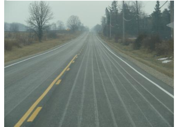
Figure 6: County's Winter Operations (De-Icing)
