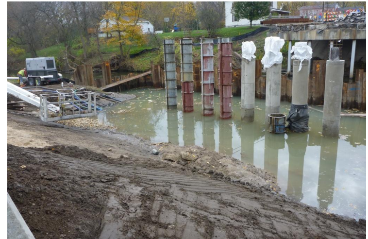
Figure 8: Pouring Piers on Blivin Road Bridge
