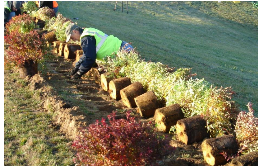
Figure 7: Installation of Living Snow Fence on Pyott Road
