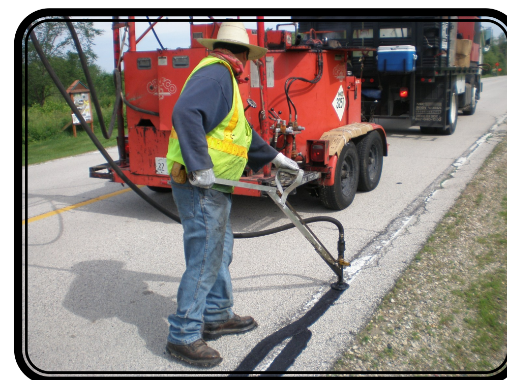
Example of Crack Sealing Treatment
