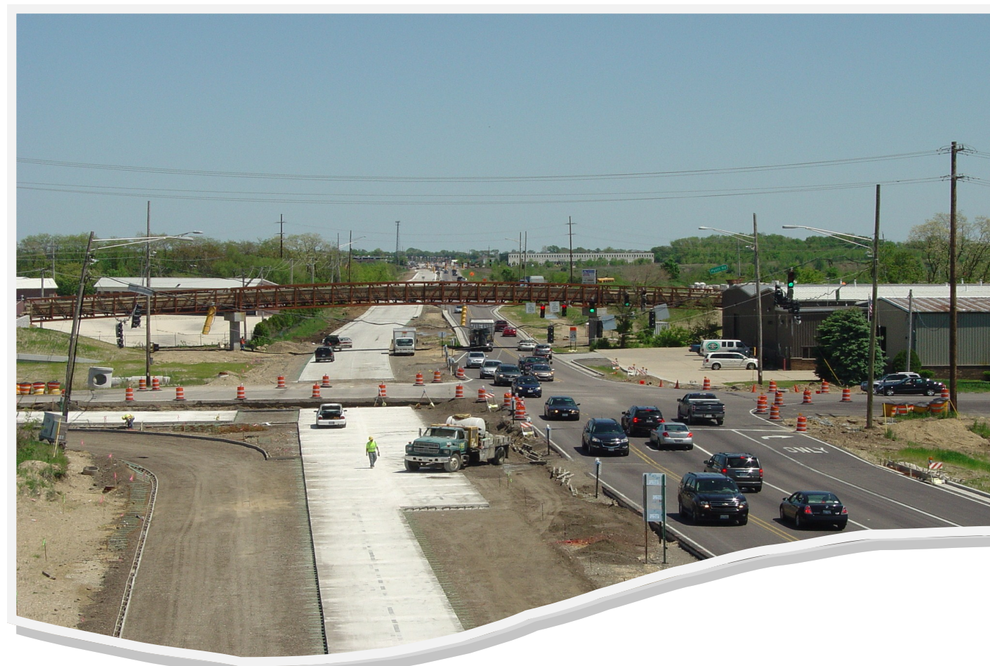
Construction of Rakow Road
