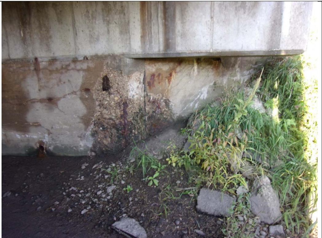
Photo 9 Northwest corner Of West abutment
