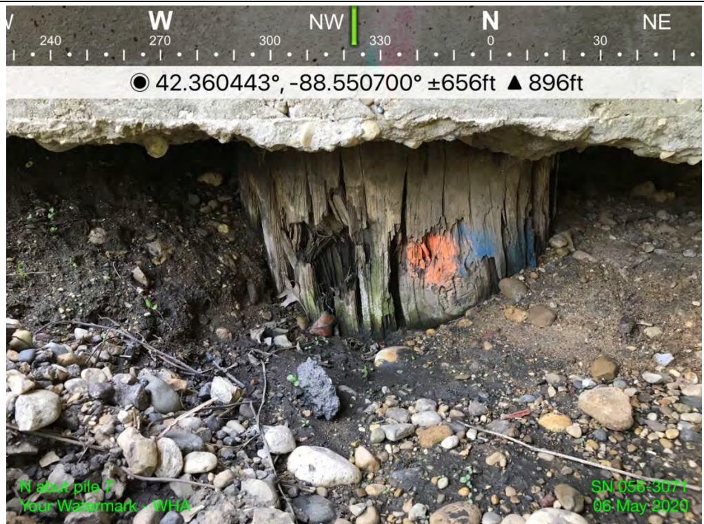
North abutment pile #7
