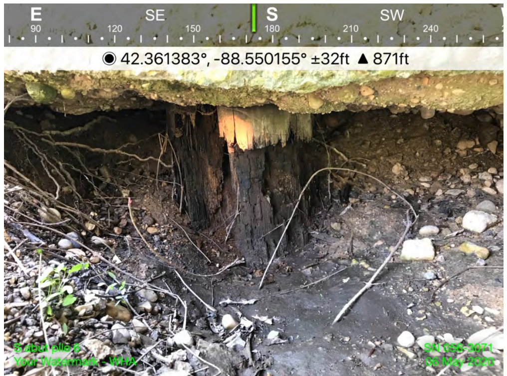
South abutment pile #6
