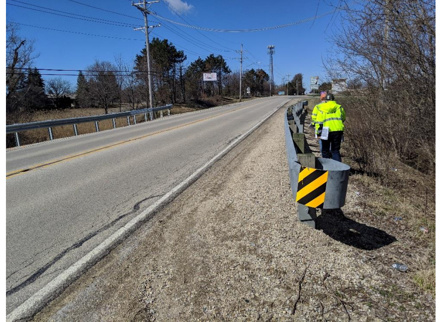
Ackman Rd, between Redtail Dr & Swanson Rd Terminals do not meet current standards.
