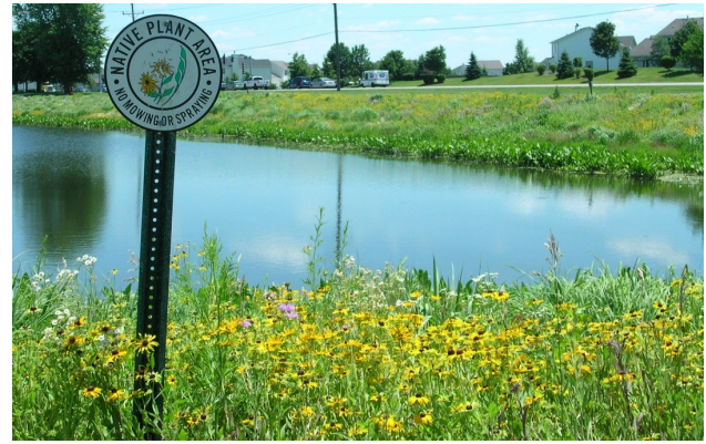
A naturalized detention basin at Montgomery Village Hall.
